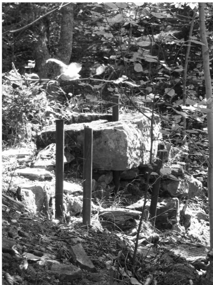
Figure 6. Remnants of the headframe foundation at the albertite mine, developed about 1870, at Albert Mines, New Brunswick.
