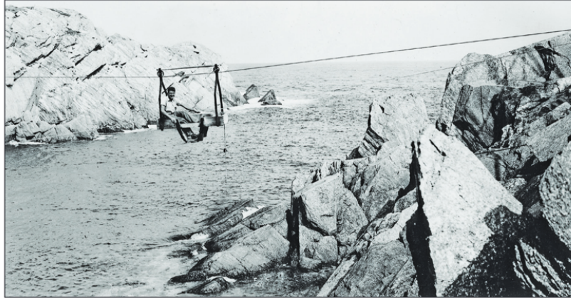
Figure 4 – The cable chair, a later installation to allow staff to transit from the main island to the north island station.
